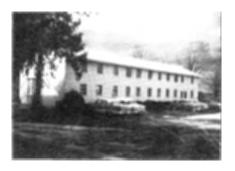
This picture of Bethel shows it as it is today, after masonite siding was placed on all of the exterior and new aluminum windows were installed. The building was completely insulated. The interior of the outside walls was paneled. New steel doors were installed and a number of other
