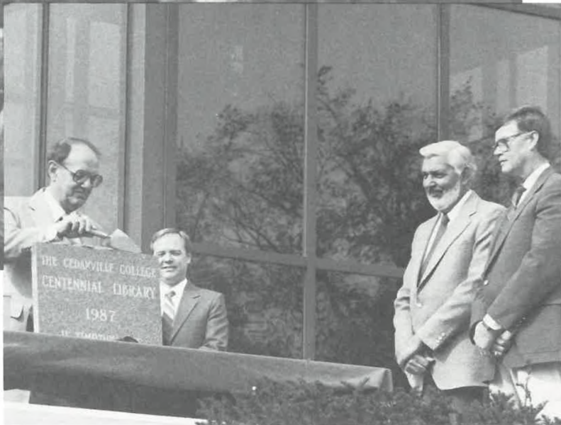
Rev. William Brock of Columbus, Ohio, Chairman of the Board of Trustees of the College, adds mortar to the corner stone of the Centennial Library. His son, Lynn Brock '68, director of library services, stands nearby.
