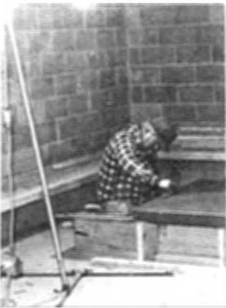
Construction worker planning.
