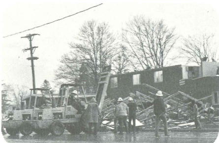
Patterson's Roof Scraped From Street
