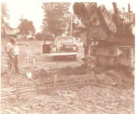
Workmen look on as ground is drilled down to bedrock for the foundation pilings.
