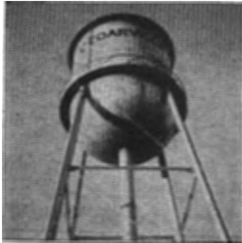
Old watertower, located at the corner of Bridge and Creamer, has to suffice for a while longer.
