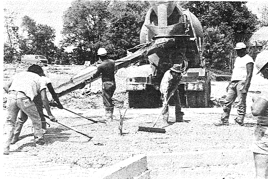
Workers lay foundation for Senior Citizens' apartments next to Leach's.
