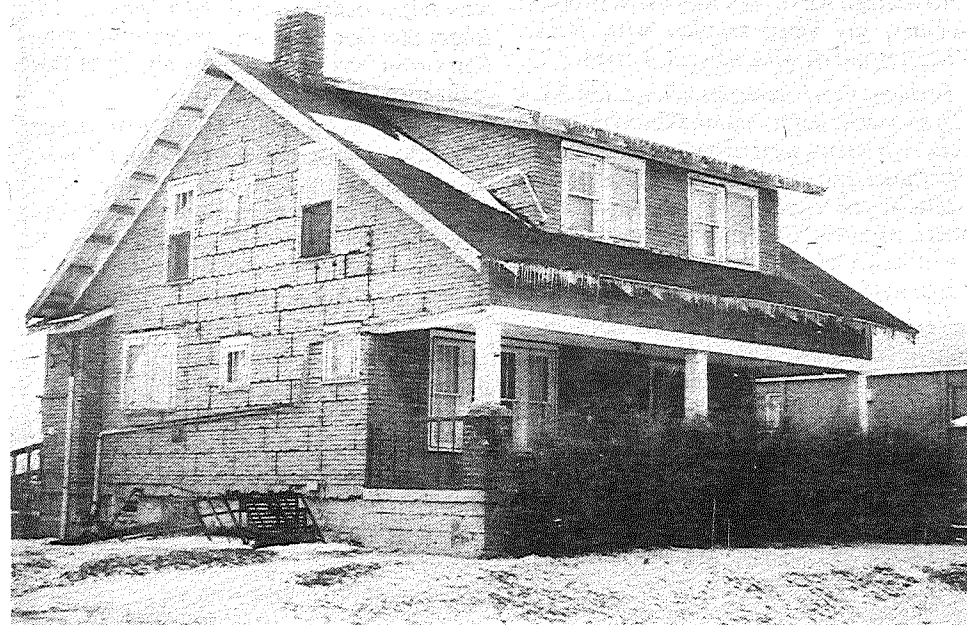
Universally ridiculed as an eyesore, implicated as a fire hazard, and questioned as inadequate, this building will remain the Cedarville College Health Service through at least 1982-83.
