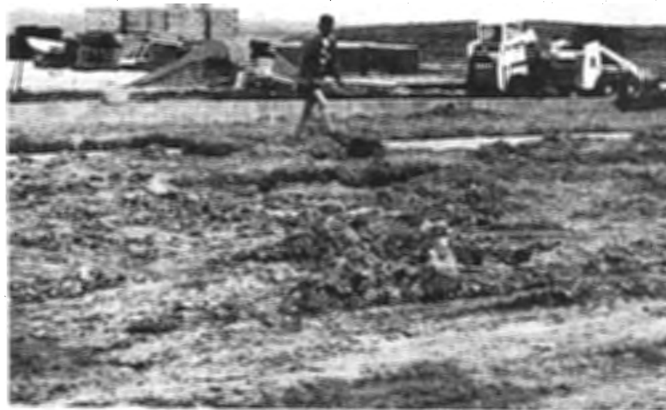
Construction on the new dormitory gets underway.
