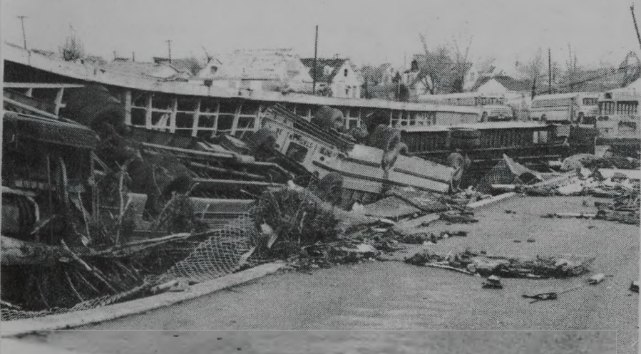
Xenia school system suffers heavy damage.
