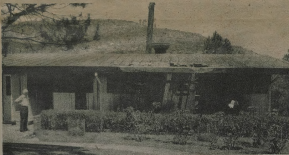
Damage done by fire!
